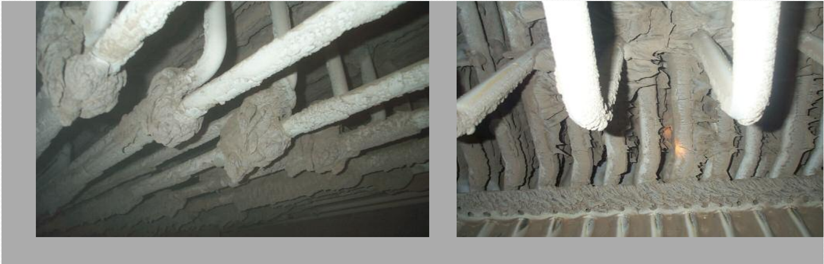
Fouling in Superheaters
