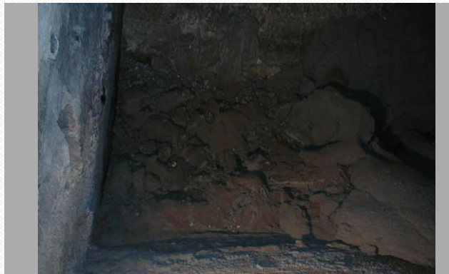
Fouling in Furnace
