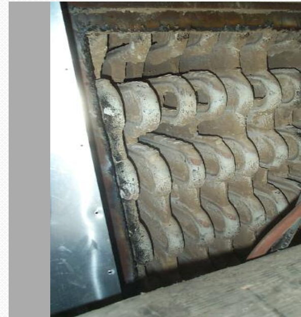
Fouling in Convective Surfaces
